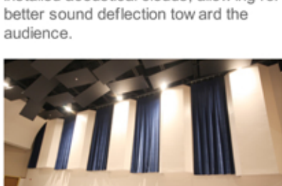
Pittsburgh Stage also designed custom curtains for the new auditorium. This included a full set of stage curtains, as well as synced, retractable, sound dampening acoustical curtains. The acoustical curtains can be extended or retracted into custom pockets with the push of a button.
